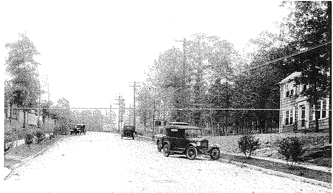
Brighton Road in the late 1920's. Note the newly planted trees.
