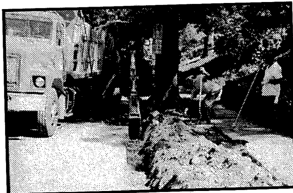
A trench is dug to prepare for a new curb.
