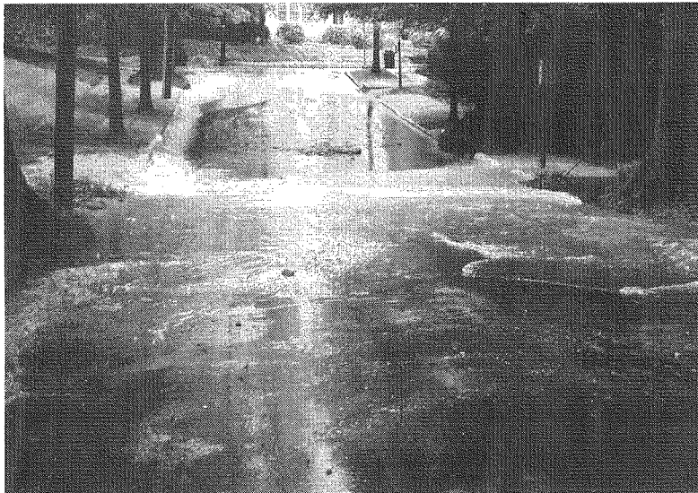
Rainwater streaming down Wakefield Drive during the June 30th storm.
